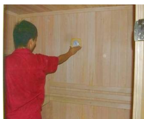
FIG-14 install the warm barothermohygrogram
