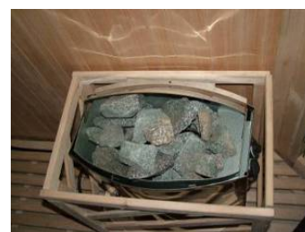
FIG-19 Place sauna stone
