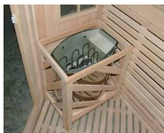
FIG-18 location of the stove
