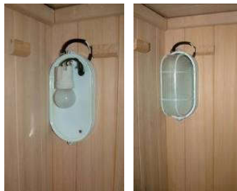
FIG-11 Assembling the light
